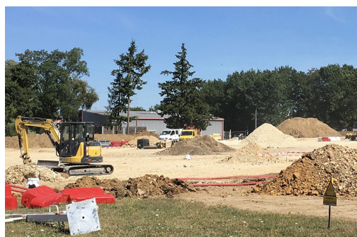
Travaux parking C7
